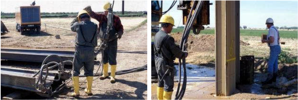
Fig. 7a/b: Trial using vibrating injection procedure
