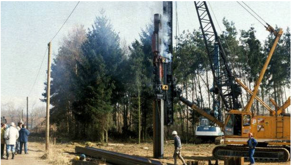
Fig. 6: Trial with classical pile driving
