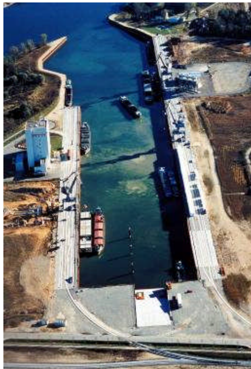
Fig. 2: Aerial photograph of the Danube Harbour Straubing in operation after completion
